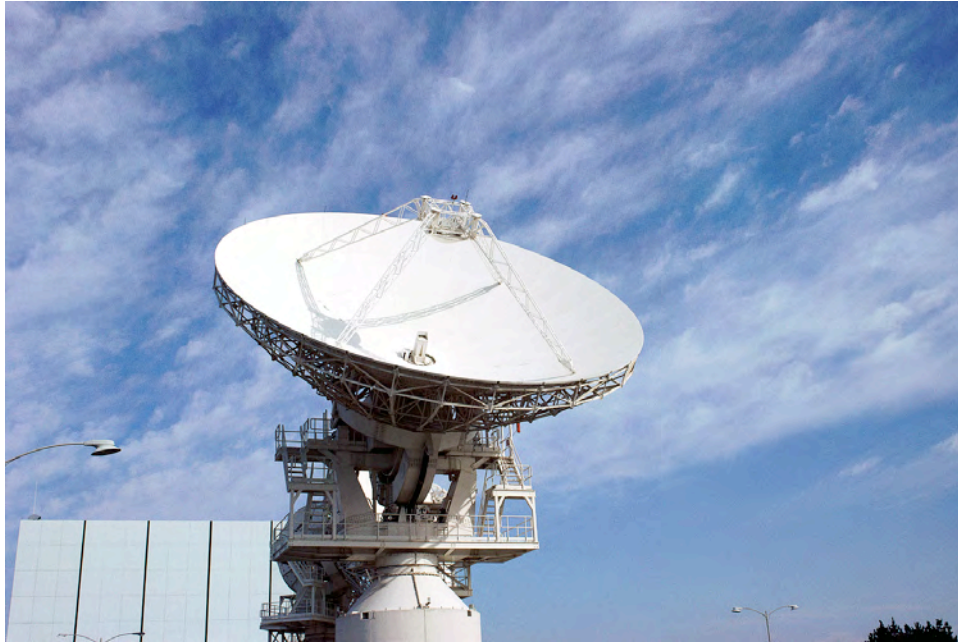
Photo 8. Fiber optics is often used to transmit data between microwave receivers and control stations to minimize the effects of EMI.
